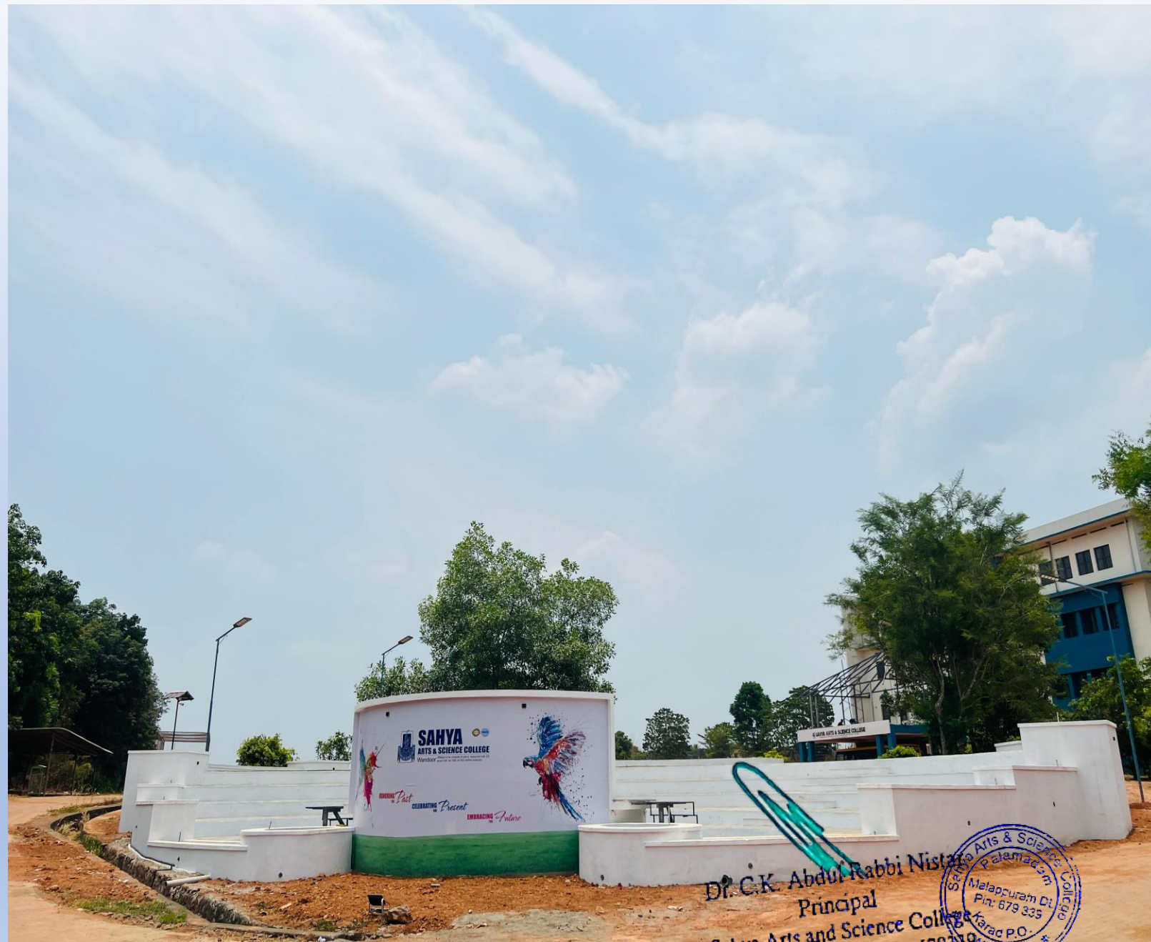
Construction of Amphitheatre
