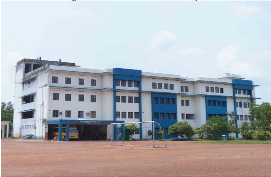
Figures -9-10 Well maintained campus
